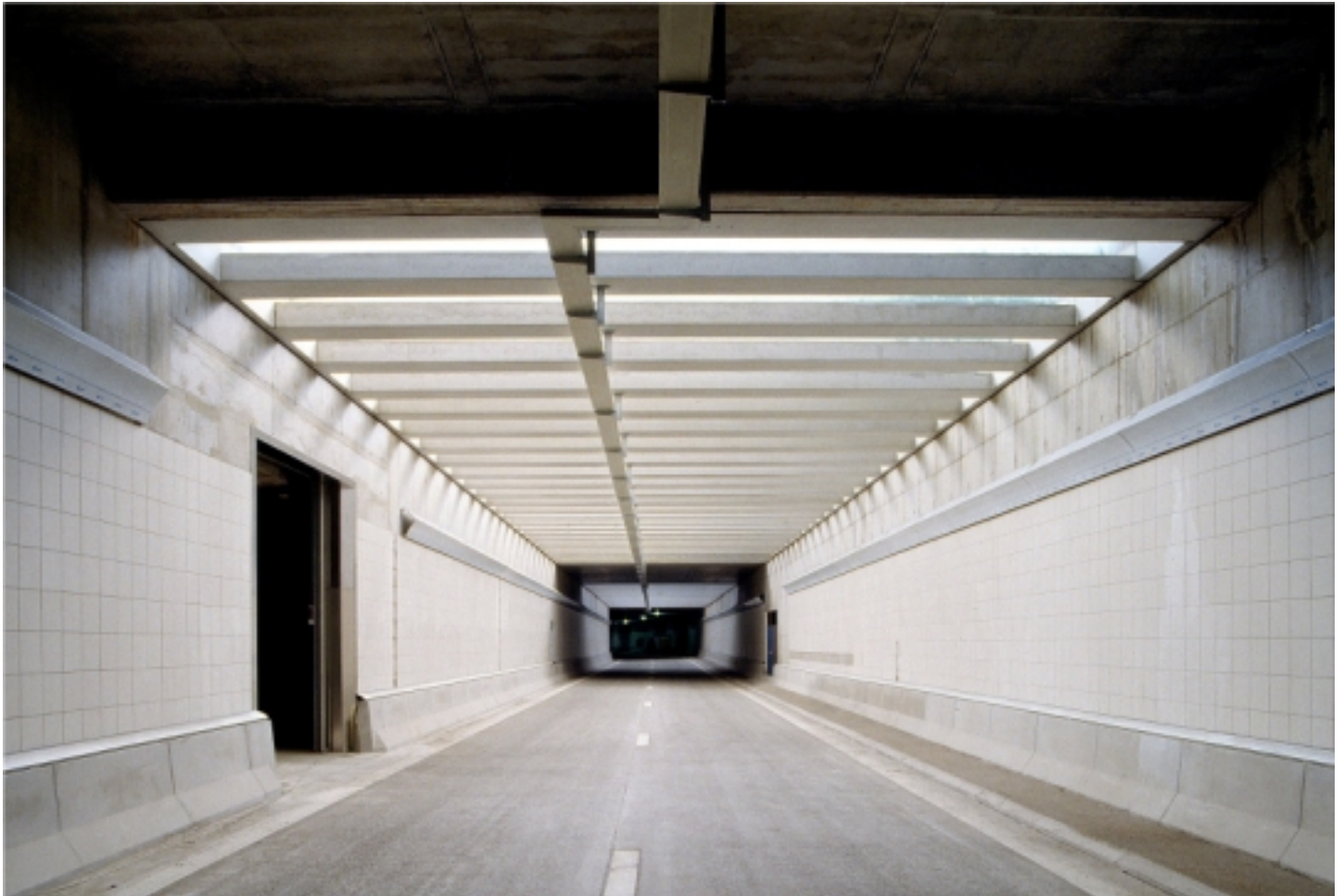
Kinkempois Tunnel (link E25-E40) in Liege, Belgium, using concrete pavement
