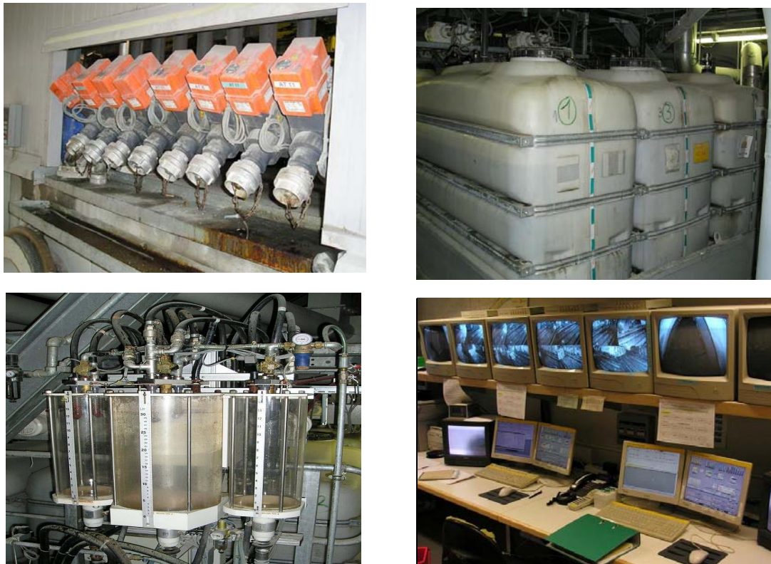
FIG. 2) Storage of admixtures in a tunnel job site in Switzerland
